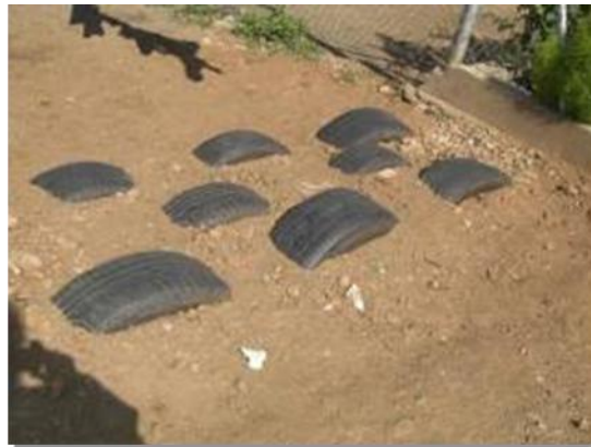
Figure 25: Completed half tire walkway
