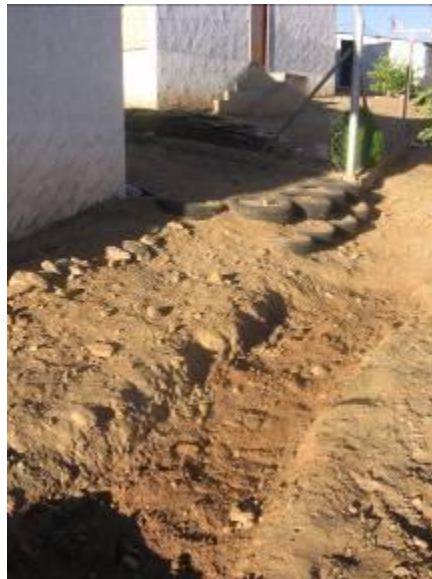
Figure 17: Completed mulch pit
