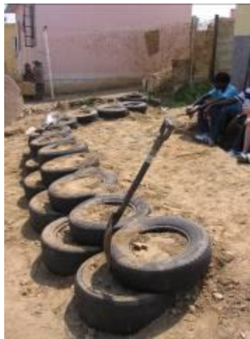
Figure 22: First completed tire wall
