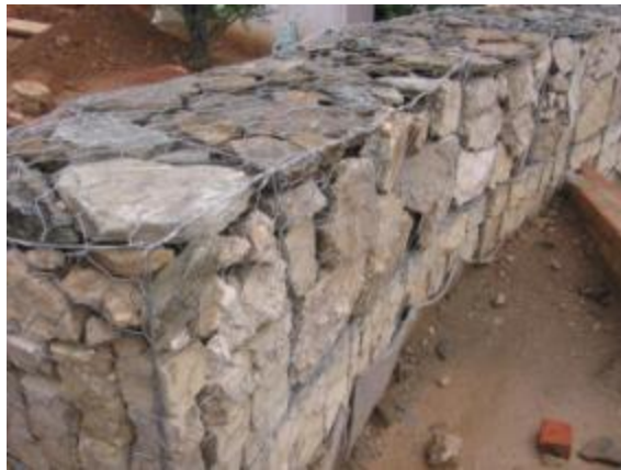
Figure 6: Gabion constructed at the HRDC in Katutura, Windhoek, Namibia
