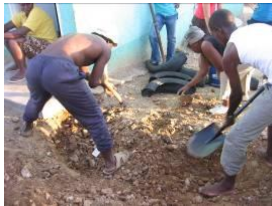
Figure 23: Digging for the half tire walkway
