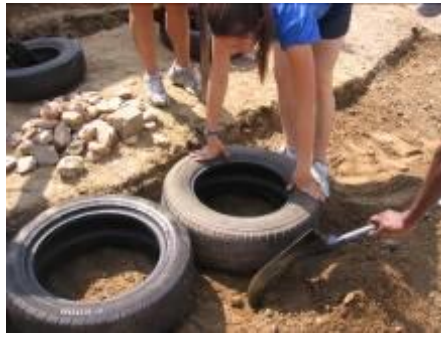
Figure 20: Placing the first row of the tire wall
