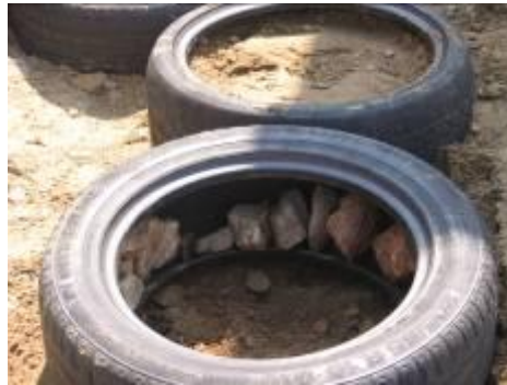
Figure 21: Filling the tires with stones
