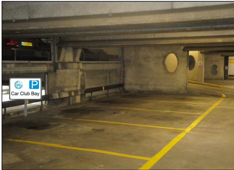
Figure B1 - Fairfield Car Park
