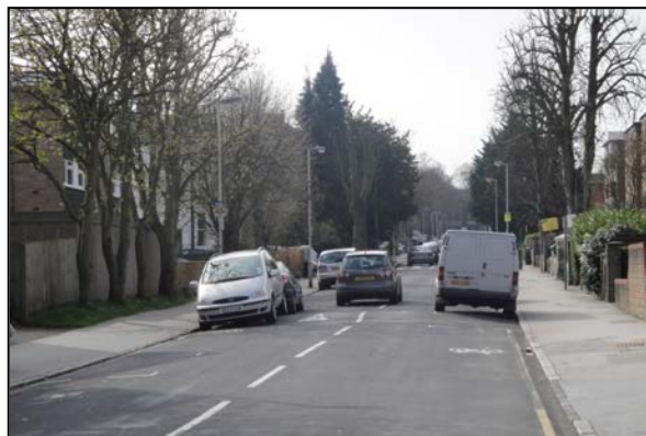
Figure 110 - Canning Road Image 2
