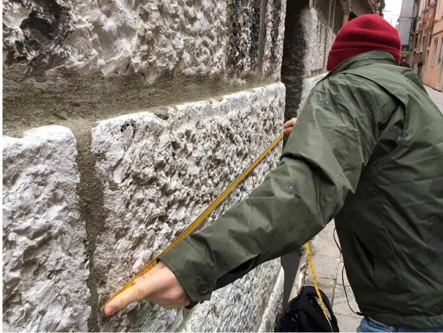
Figure 16 - Measuring the exterior blocks of the bell tower base
