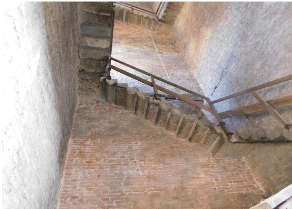
Figure 58 - Interior of Carmini to illustrate why the railing is important
