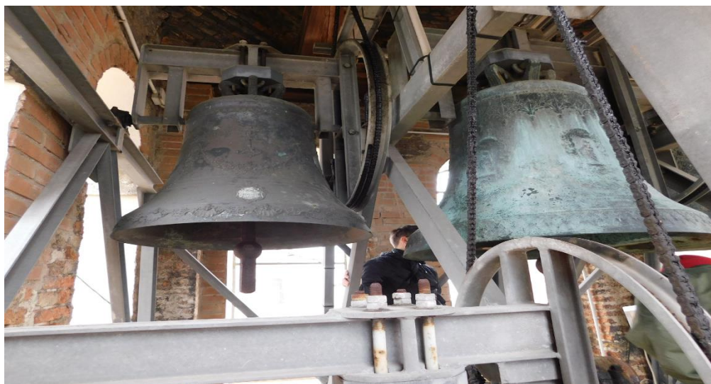
Figure 25 - The sonello(L)is the smallest bell and not tuned to the scale of the rest of the peel.
