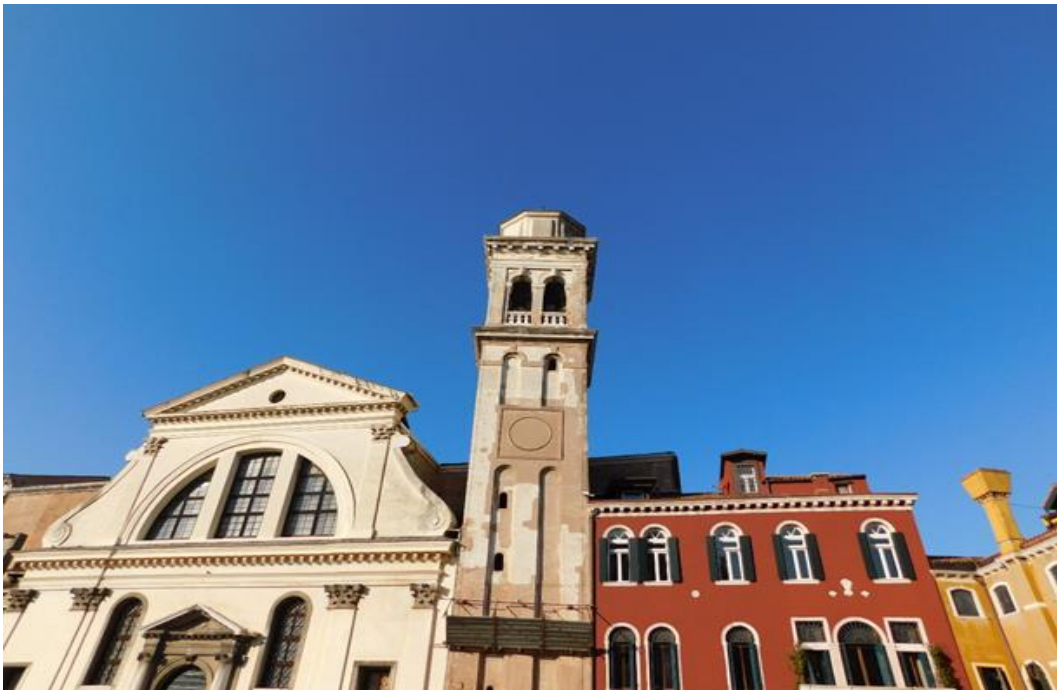
Figure 53 - San Trovaso leaning to the right
