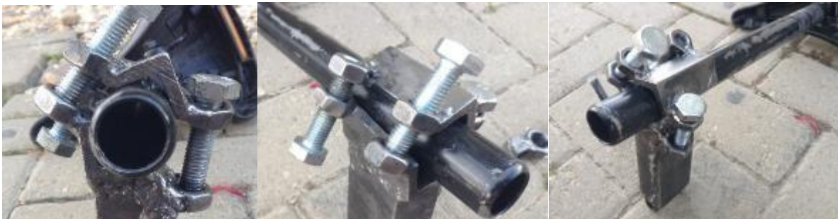
Figure 62: Angle iron properly lined up
