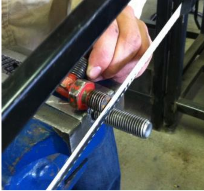
Figure 52: Cutting the bolts with a hand saw
