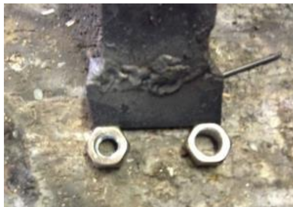
Figure 60: Lining up the hex nuts on the angle iron
