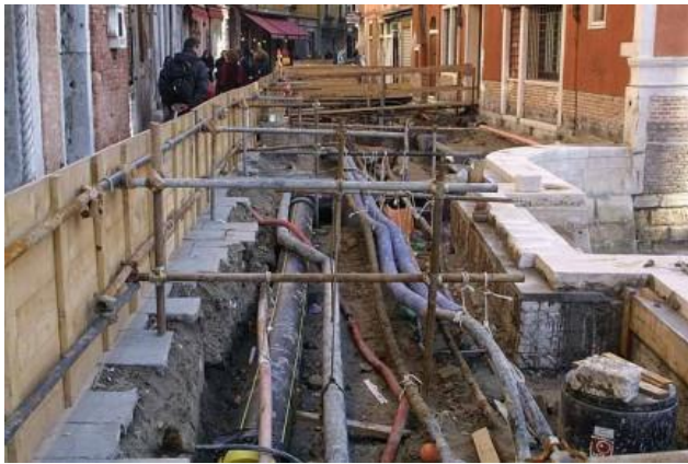
Figure 5: An Insula maintenance project of the utilities under a walkway
