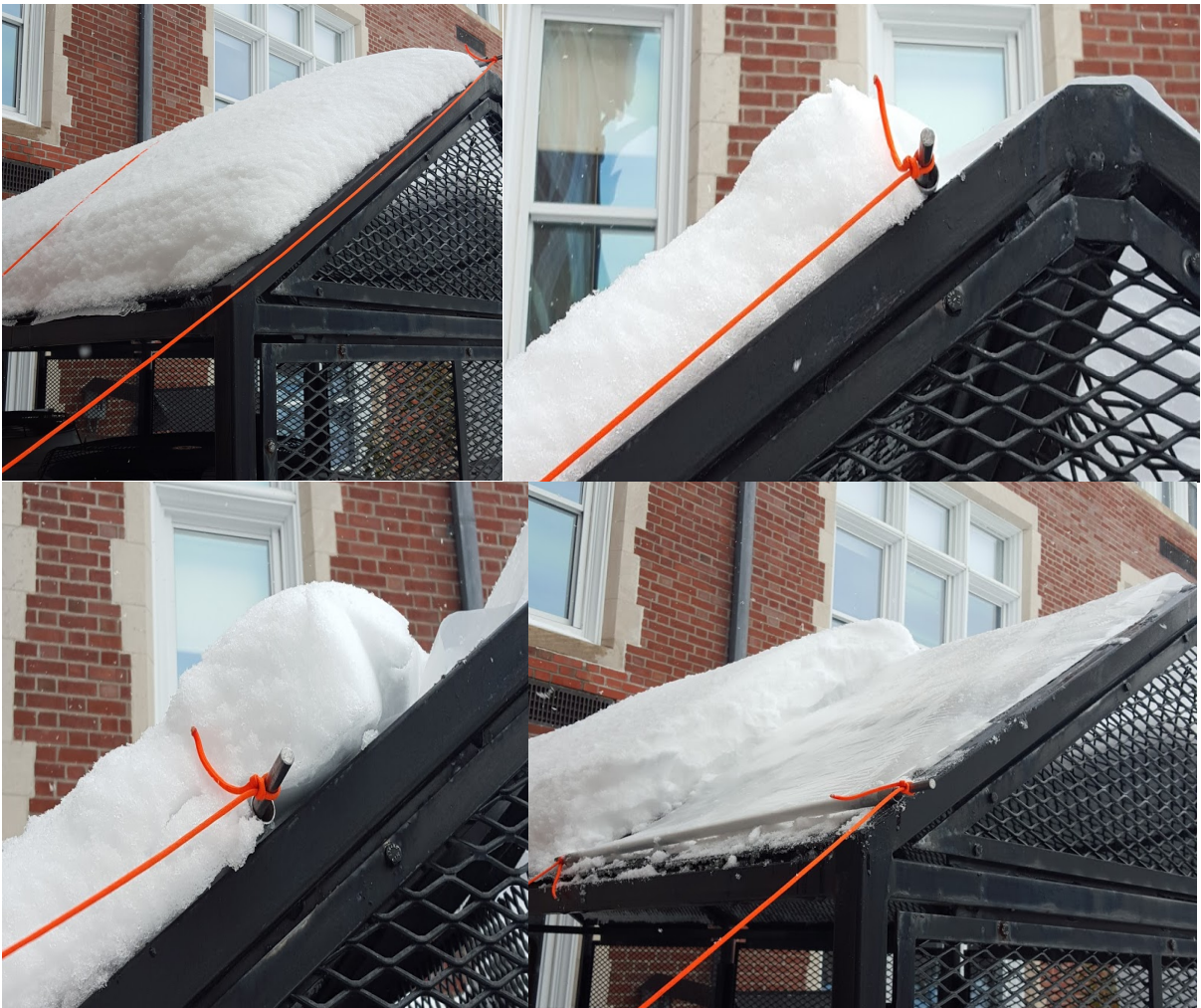
Figure 60: Tarp Roller Roof Clearing
