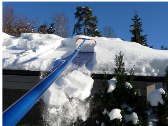
Figure 8: Advanced Roof Rake Clearing Snow
