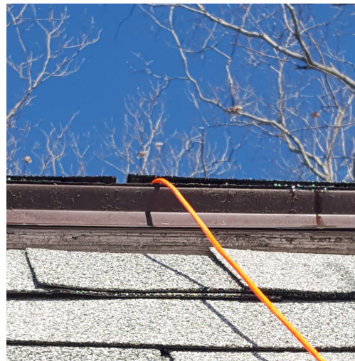
Figure 57: Rope Caught Under Shingles
