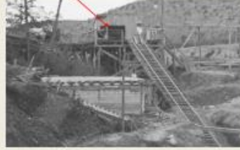
Power Assisted Car Hoist to 50 Feet Depth
