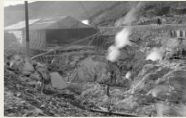
Removing Unsuitable Granite at Section 3
