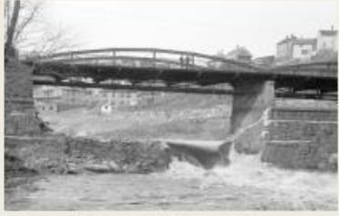
Downed Lancaster Mills Dam 1897
