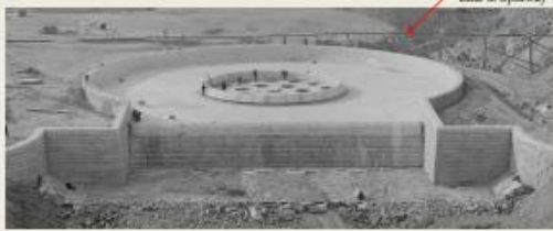
Pool, Weir and Erosion Control Apron 12.01.1903
