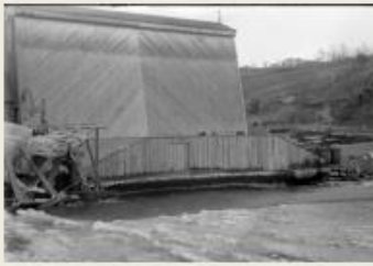
Flume Intake at Springtime High Water
