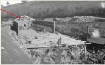
Flume, Section 4 built before Section 3
