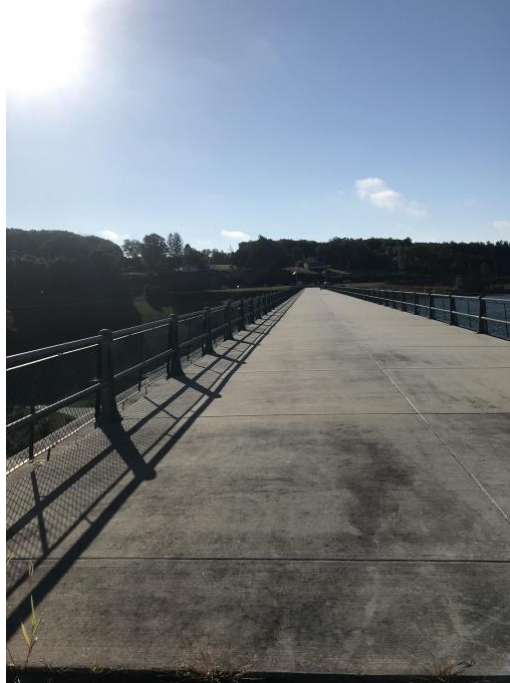
Figure 45: On Top of the Dam
