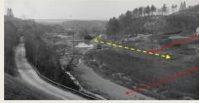
Drained Lancaster Mills Pond
