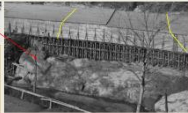
High Granite Profile Cleaned Before Building the Flume
