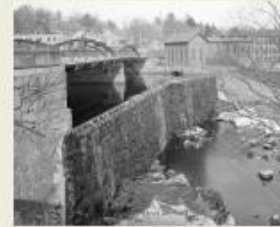
Lancaster Mills Dam
