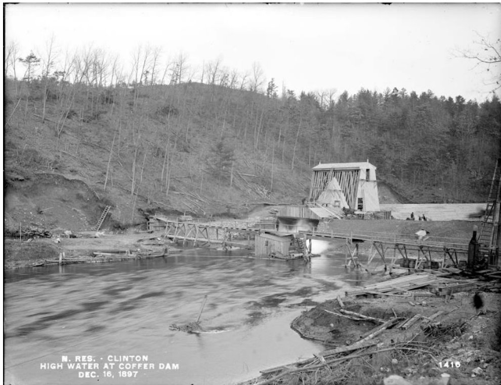
Figure 5: Picture 1416: (Dec 16, 1897) from Photograph, Wachusett Dam Construction, June 20, 1898: Exhibits: Institute Archives & Special Collections. (2003, July).
