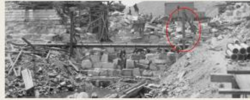
Lancaster Mills Supply Pipe Rerouted through Lower Gate Chamber
