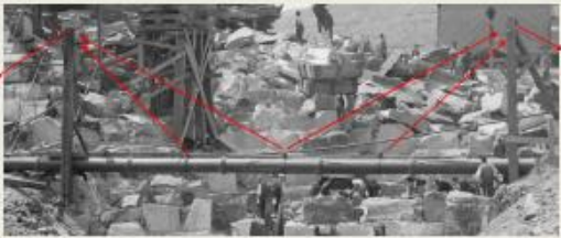
Lancaster Mills Supply Pipe – Support Masts
