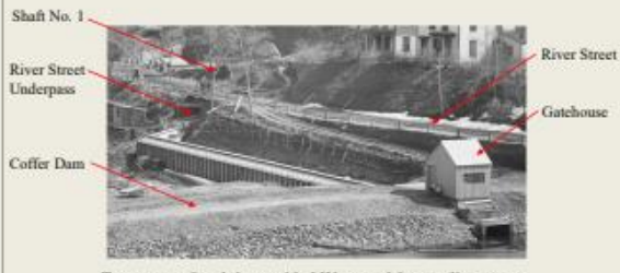
Temporary Conduit provided Water to Metropolitan Area
