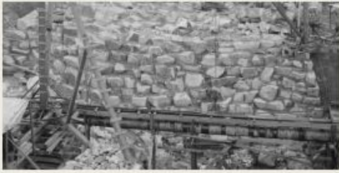
The Flume Gap and the Lancaster Mills Supply Pipe
