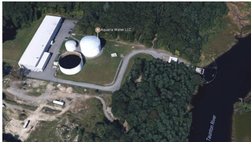
Figure 3: Aerial view of Taunton River Desalination Facility (Google Maps, 2017)
