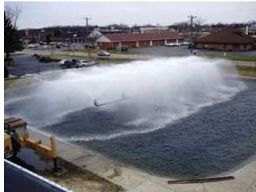
Figure 2: Floating Spray Coolers at a Paper Mill in Pakistan.
