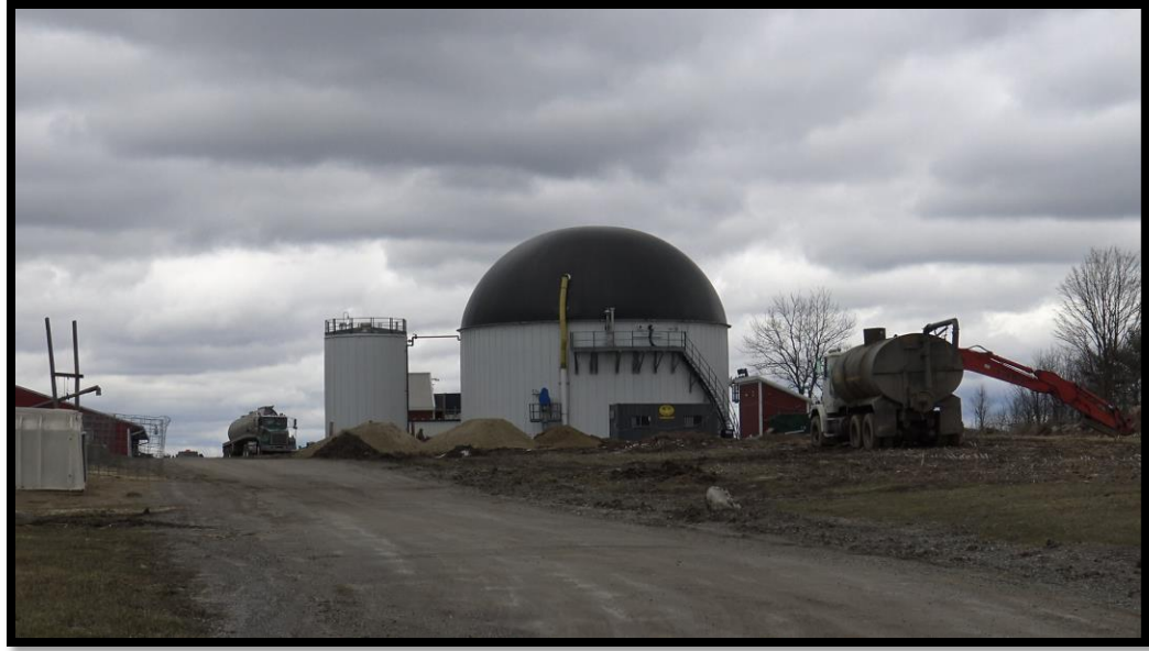
Figure 4: Photo Image of Jordan Dairy Farm's Anaerobic Digester This figure shows an example of an anaerobic digester situated on a dairy farm.
