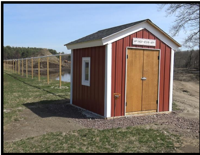
a.) Perimeter Vapor System Shed and Fence
