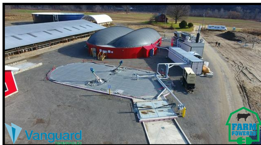
Figure 14: Drone Image of Anaerobic Digester at the Bar-Way Farm Inc. in Deerfield, MA This figure shows an example of an anaerobic digester situated on a dairy farm.
