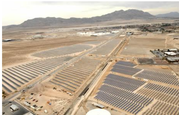
Figure 6: Nellis Air Force Base Solar Panels (Source: http://www.metaefficient.com/news )
