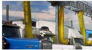
Figure 3 - Trucks plugged into IdleAire (2008)
