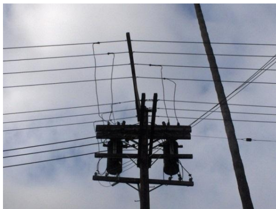
FIGURE 2 - OVERHEAD TRANSFORMER [2]
