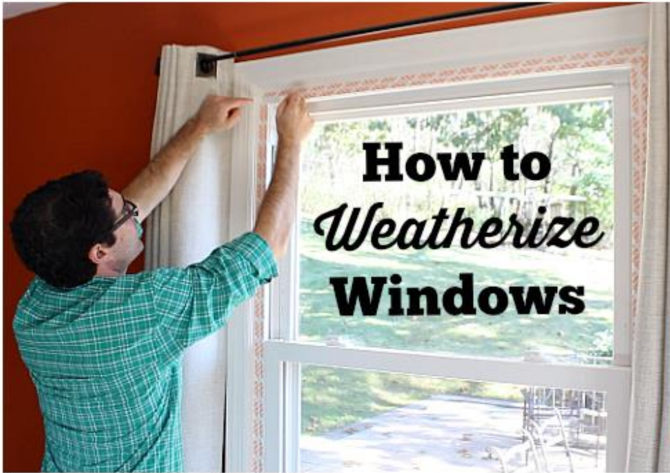
Figure 10: Weatherizing windows with Plastic Film insulation. http://www.homerepairtutor.com/how-to-weatherize-windows-with-plastic-film-insulation/ . (Patterson, 2014).
