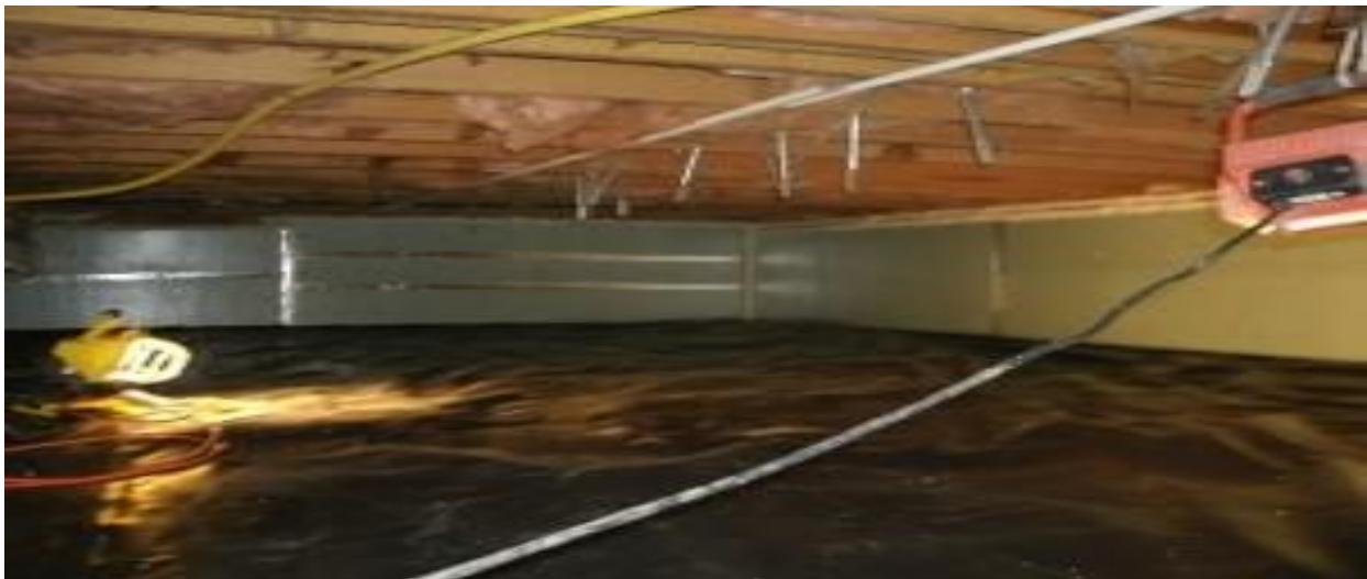
Figure 12: The aftermath of a crawlspace treatment procedure (after weatherization). http://edge-gogreen.com/home-performance/home-performance-and-weatherization/crawlspace-weatherization/ . (EDGE Energy, 2015).
