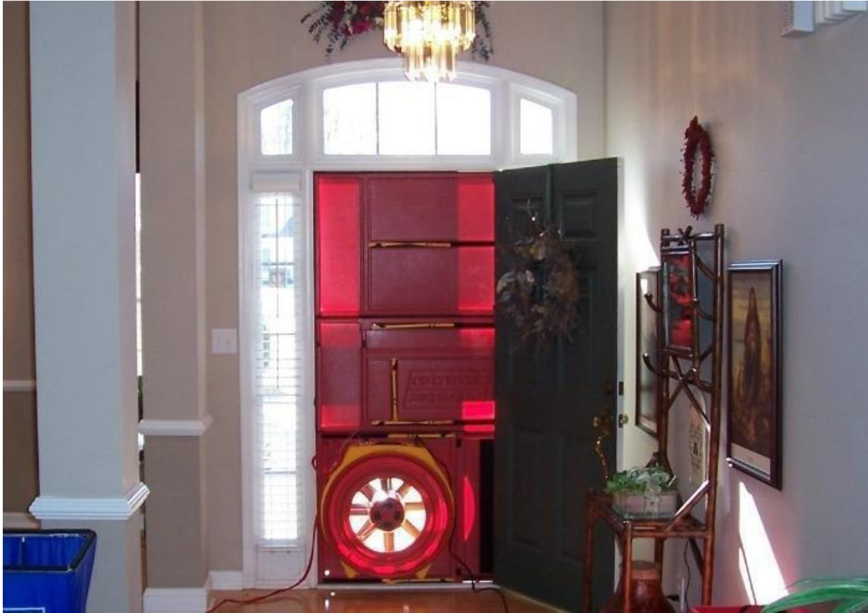
Figure 3: Blower door test during a home energy audit. https://www.holtkamphvac.com/ . (Holtkamp Heating & A/C, Inc., 2012).
