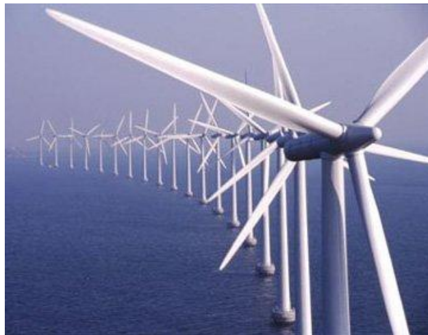
Figure 26: Offshore Wind Farm 69
