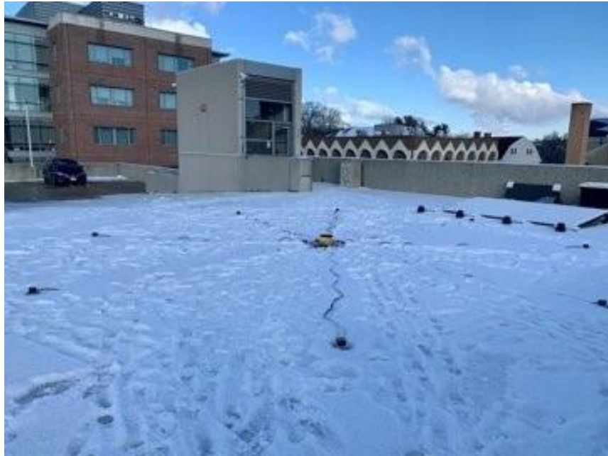
Figure 22: Field testing conditions on Roof of East Garage
