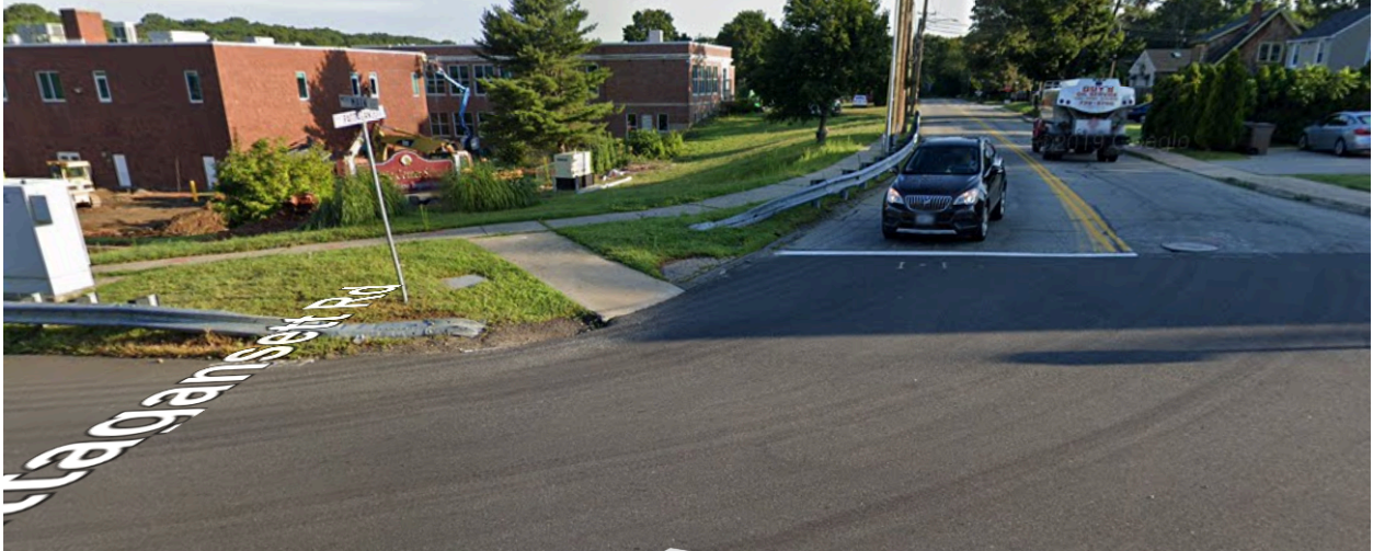
Figure 42: Google Earth view of Existing Condition of Curb Ramp i at Intersection A.
