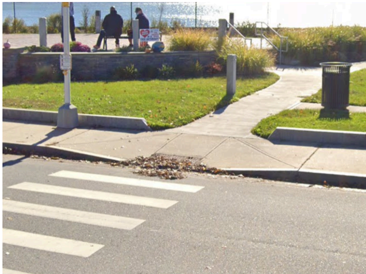
Figure 46: Google Earth view of Curb Ramp i at Intersection I.
