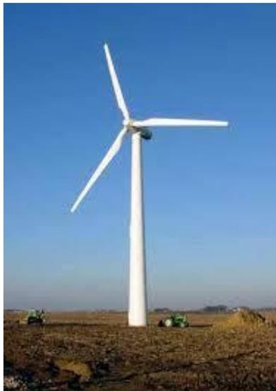
*Figure 4: Horizontal axis wind turbine*
