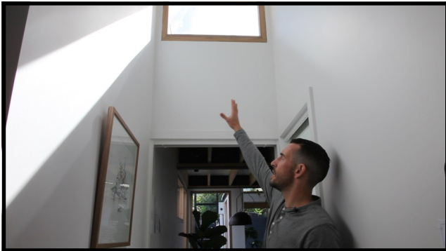
North facing windows used for light and passive heating
