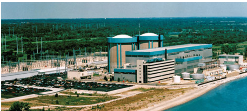
Zion Nuclear Power Plant in 1997
