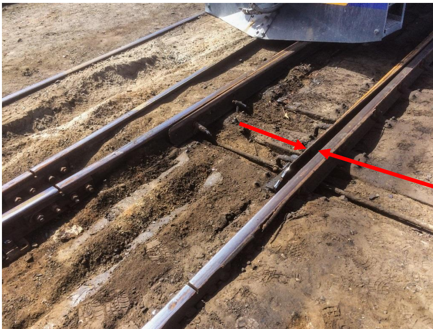
Figure 10 Picture of "halfcocked" point causing derailment
