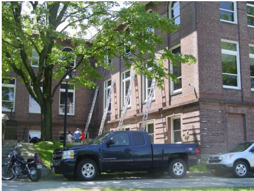
Figure 6.6: Exterior Photograph of Atwater Kent Laboratories showing the west wing
