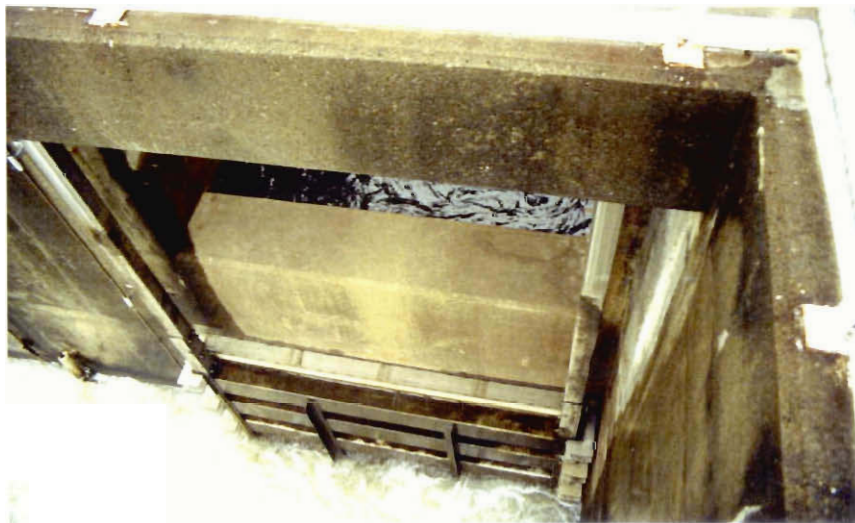
Figure 8: Sluice Gate at Vermont Yankee Nuclear Power Corporation
