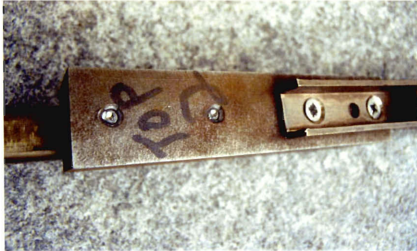
Figure 17: Bronze Covers on Tongue of Sluice Gate
