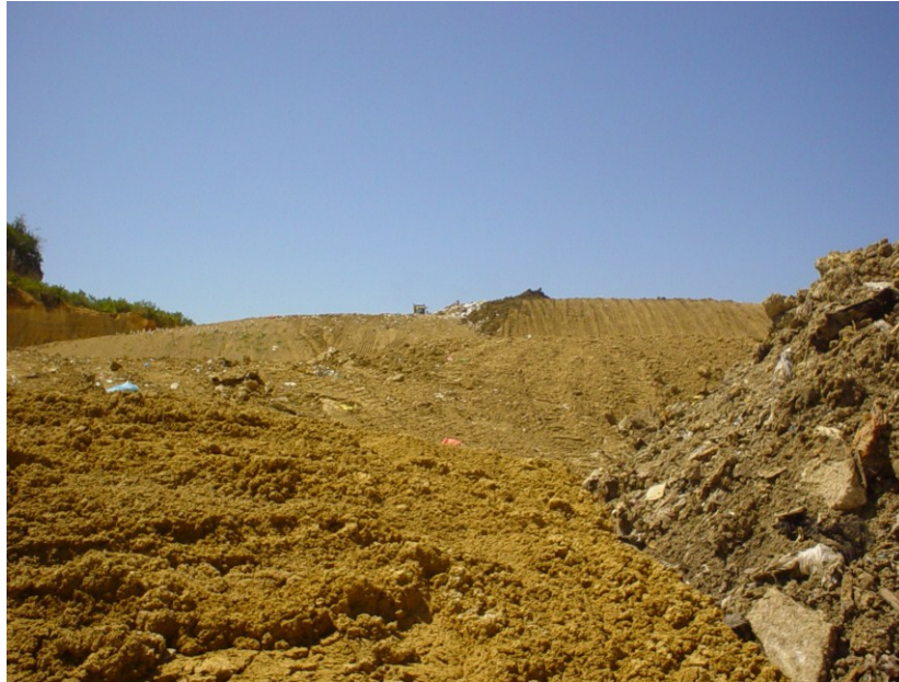
Figure 13: The Yauco Municipal and Industrial Landfill
