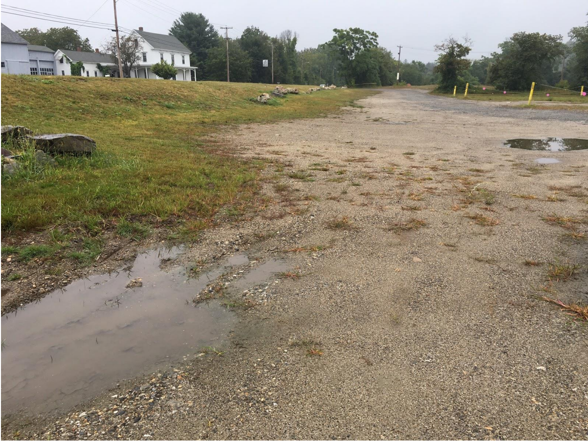
Figure 4.13: This figure shows Lot A (right), and how it rests at a lower elevation than Main St (left). Main St. runs parallel along the top of Lot A and disposes stormwater runoff down the sloped hill and onto Lot A of Ski Ward Hill.
