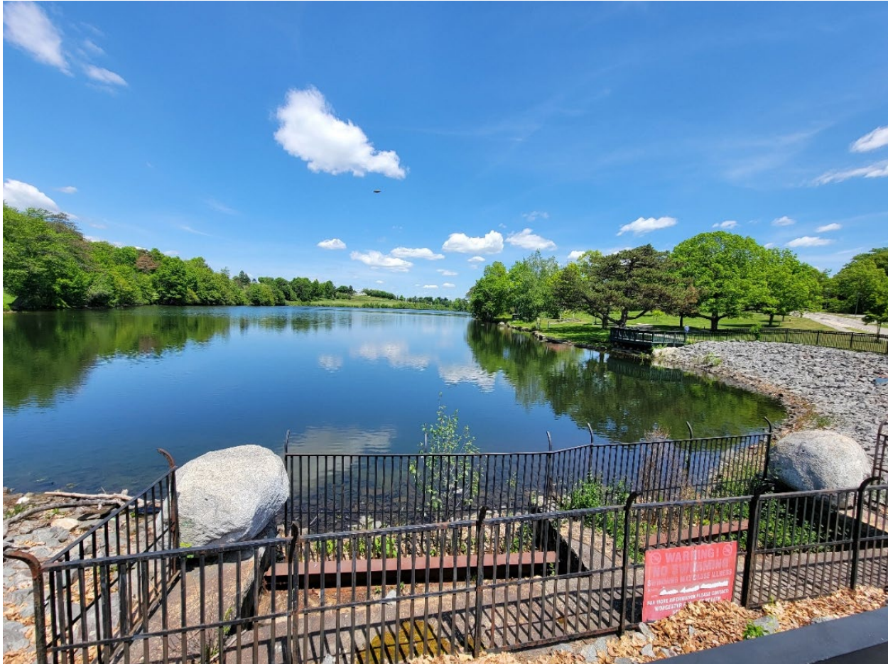
Figure 8: Image of Dam at Green Hill Pond
