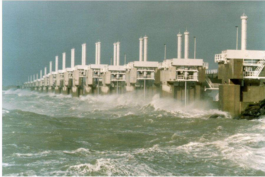
Figure 7: Movable Gates in Holland
