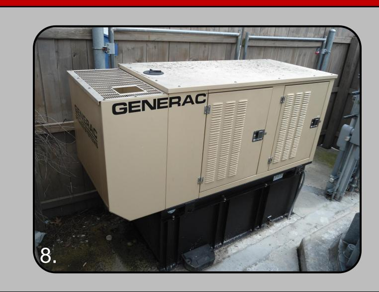
Backup generators assist with long term backup power, but startup times are longer than both batteries and flywheels and thus cannot act as a buffer to electrical instability. Valve Regulated Lead Acid batteries (VRLA) and flywheel systems can work with generators to mitigate startup times.
