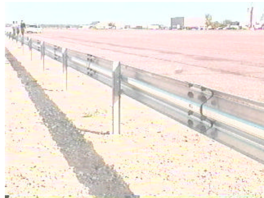
Figure 49: Guardrail installation of a modified G2-system with splice connection between posts.
