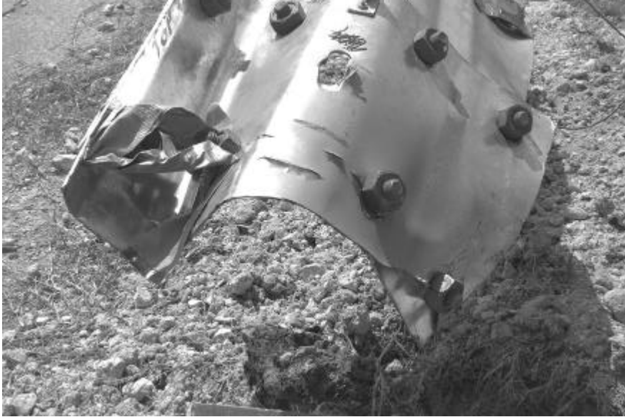
Figure 6: Ruptured rail element at splice in TTI Test 405421-2. (16)
