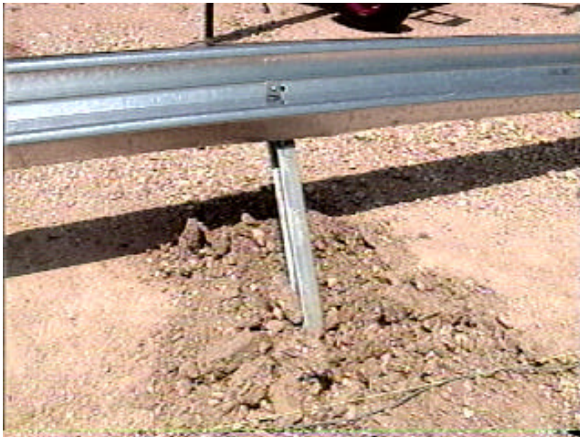
Figure 105: Post-test close-up on post.
