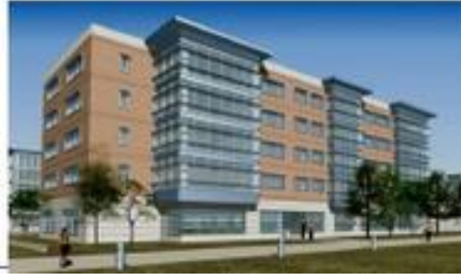
Figure 4: East Hall—horizontal sun-shading
