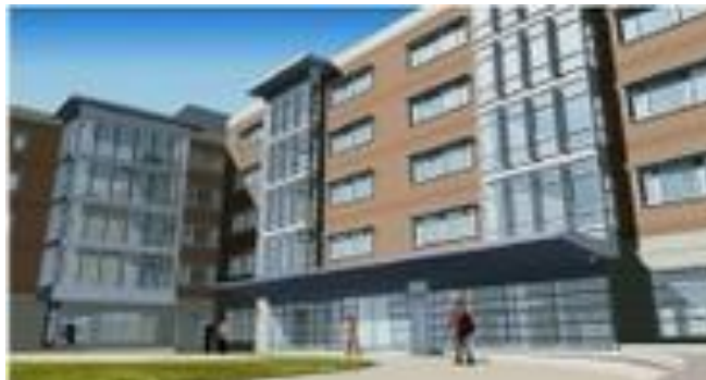
Figure 3: East Hall—vertical sun-shading
