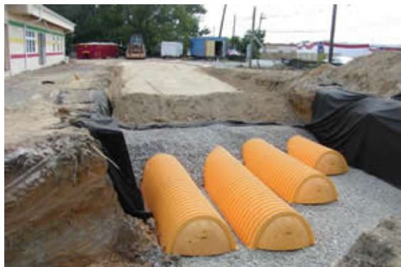
Figure 3-StormTech Chambers (StormTech, StormTech SC-740 Chamber )
