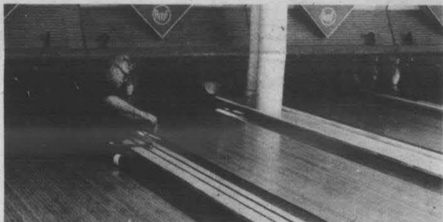
Earl Reagan begins repairs on damaged lanes.
