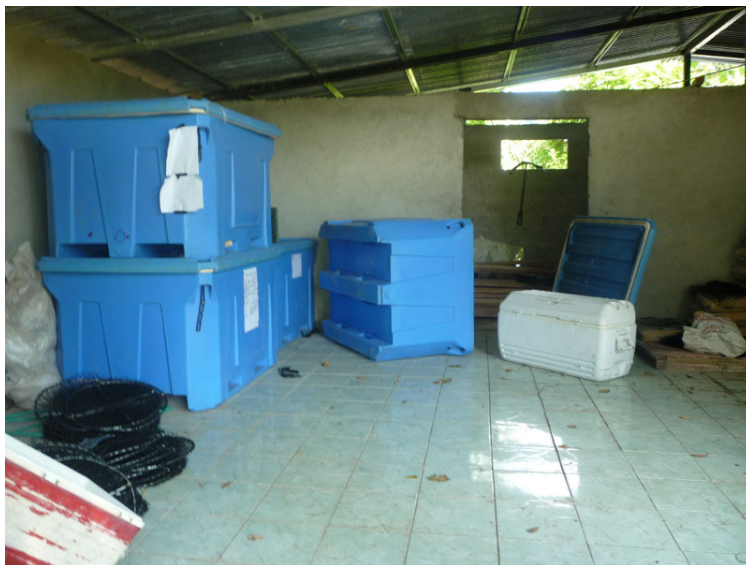
Figure 15: The fish processing center currently being built at ASOPECUPACHI headquarters.
