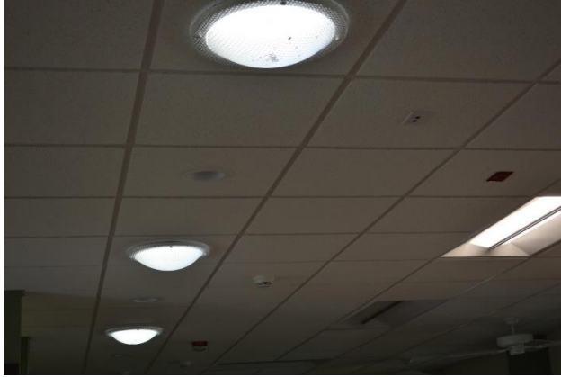
Figure 8. Passive solar domes (left) contrasted with electric lighting (right) at EARTH University
