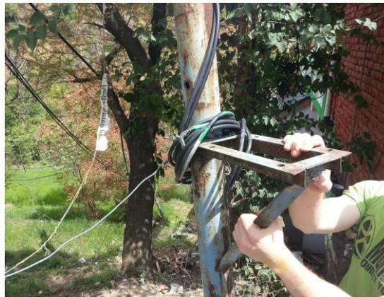
*Figure 1. A broken solar street light with a missing battery*
