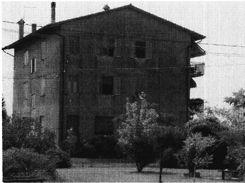
Figure 36: A Moderna Non Intergrata Building
