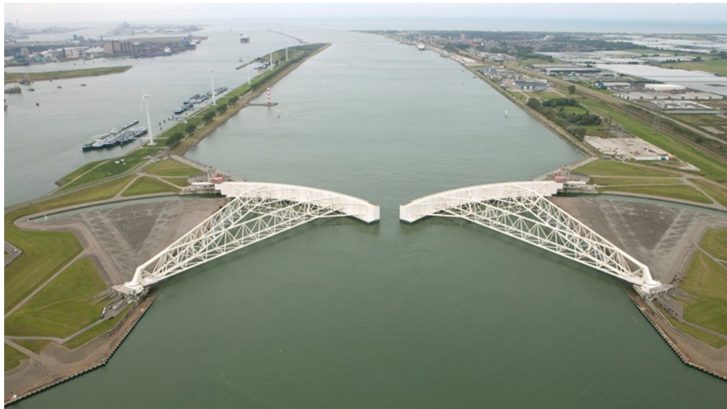
Figure 4: Maeslantkering in Rotterdam (ANP, 2018)
