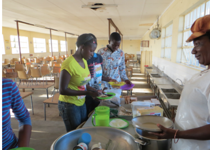
Figure 10: Students being served breakfast at the cafeteria. The broken sinks can be seen lining the walls to the right and there is significant ceiling damage. Source: Tauno Iipinge, used with permission from EduVentures
