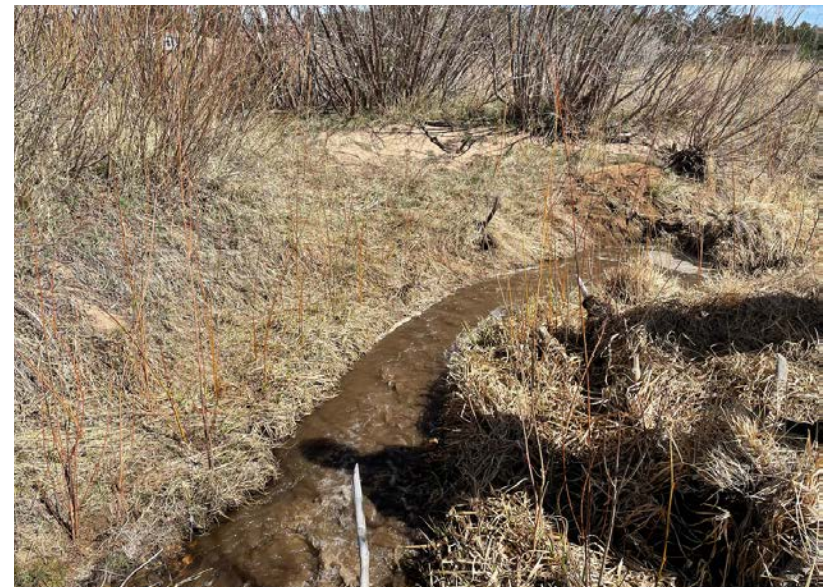
Figure 3.13: Staked willows on the bank of the Fish Creek site. Photo taken by Michael Beskid.
