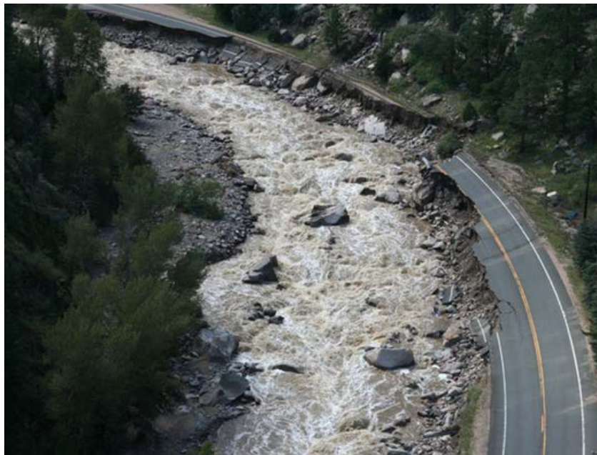
Figure 2.8: The Big Thompson River flooding and breaking nearby U.S. 34 (Lafley).
