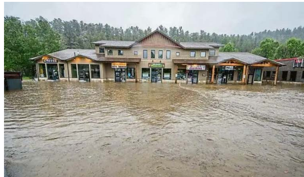
Figure 2.6: East Elkhorn Avenue flooded from 2013 (Messal).
