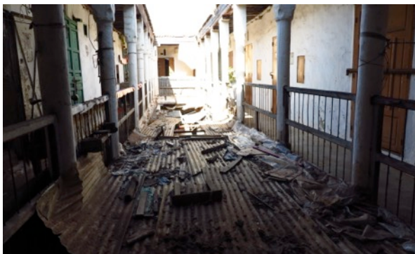
Figure 37 First Floor roof of Ben Aissa
