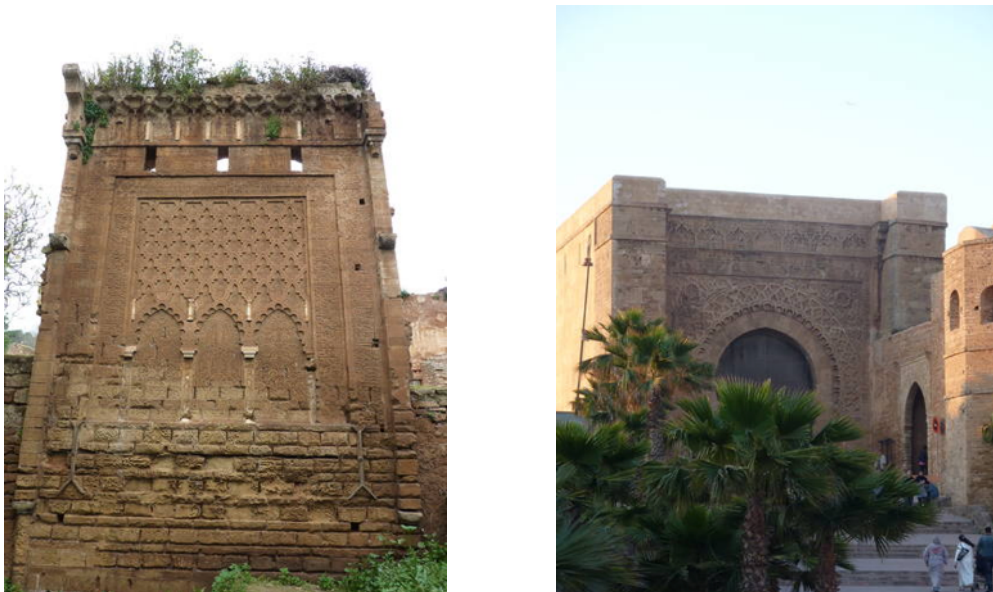
Figure 3 & 4: Finished restoration of the Kasbah of the Oudayas and Chellah (Rabat, 2012)
