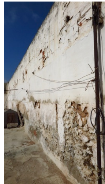
Figure 17. Wall of foundouk Jdilda
