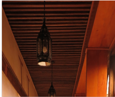
Figure 16. Roof of the Nejjarine
