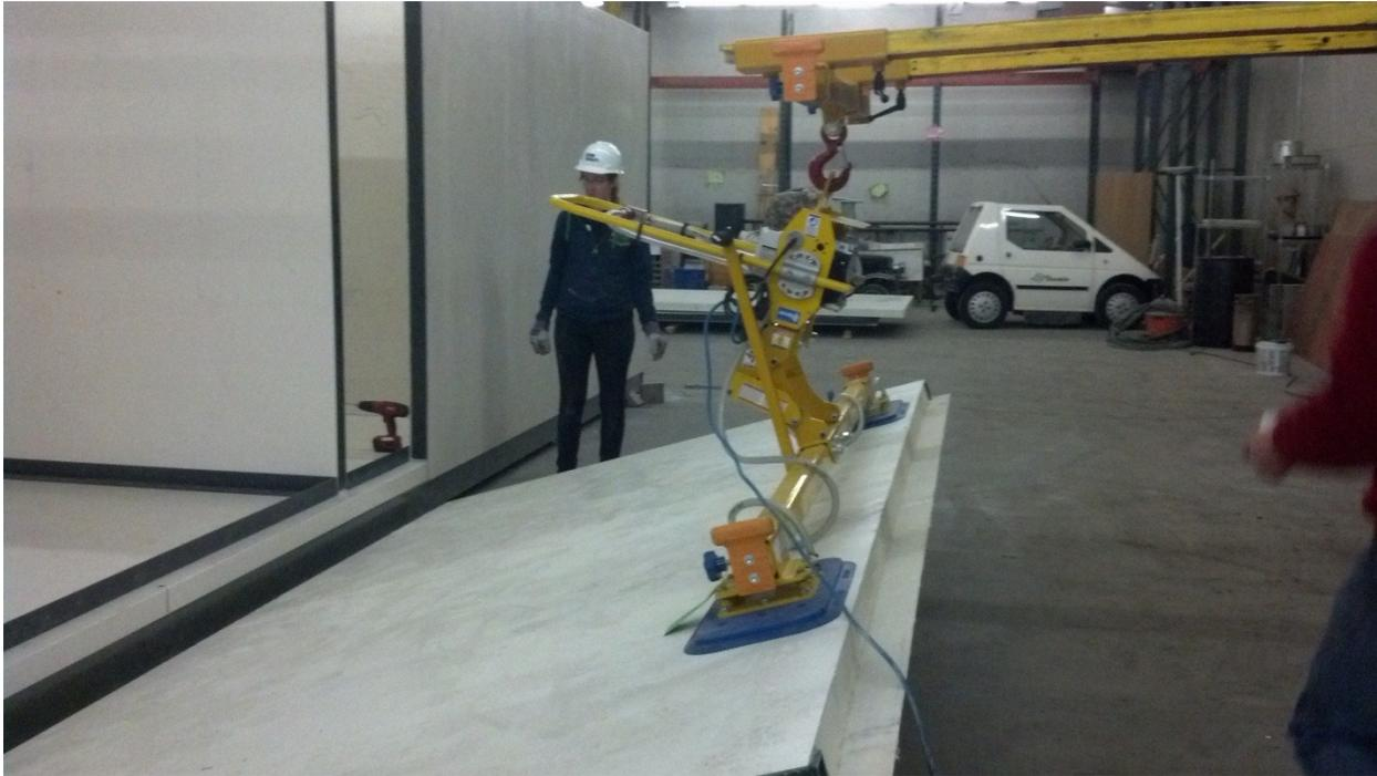
**Figure 49** Photo of vacuum lift forklift attachment used to place a wall
