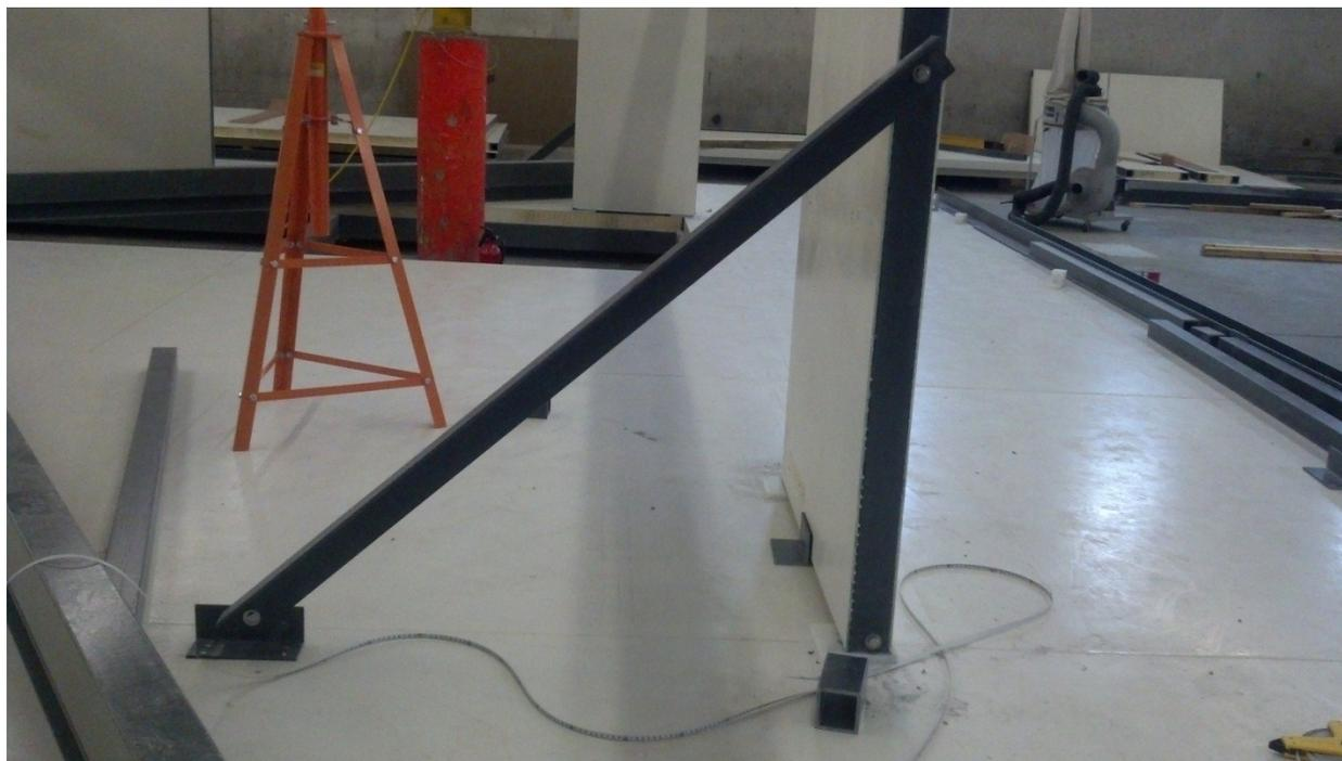
Figure 50 Photo of FRP angle being used for wall bracing
