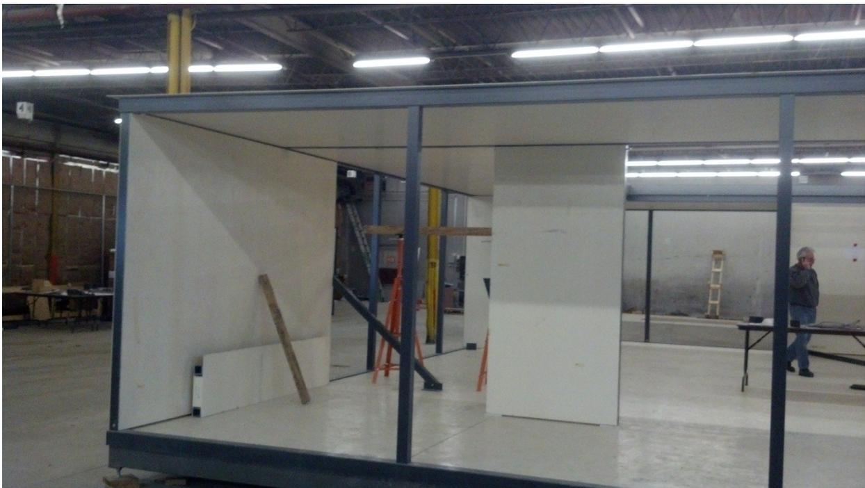
Figure 60 Photo of Solatrium practice build after one of the roof panels have been connected.
