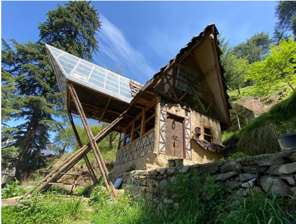
Figure 21: The Dhajji cabin designed and constructed by NORTH Architecture Firm in Naggar. The wooden lattices with stone inlays and mud plastering can be seen indicative of traditional construction with a modern form.
