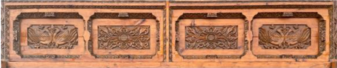
Figure 12: Image of an exterior façade to the Tara Devi Temple in Shimla, originally built around 1766, it was recently renovated/reconstructed from 2015-2018 upholding as close to the original style. The precision of detail in symmetry and form is to be noted, with perfect repeated motifs of flowers, leaves, geometric shapes, and peacocks.
