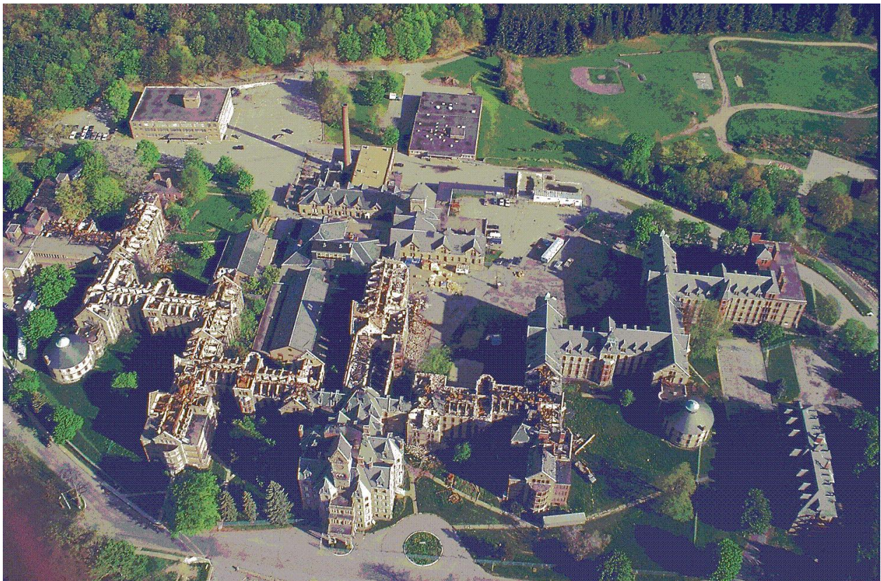
Figure 2: Worcester State Hospital after the 1991 fire (Gilbane Building Company, n.d.)
