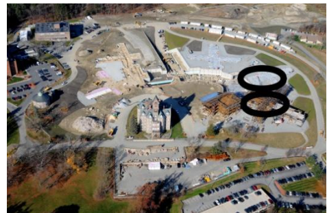
Figure 13: Areas of the construction site where cracks were found in A Wing (bottom circle) and B Wing (top circle) in November 2009.
