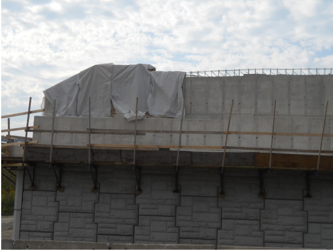
Figure 97: Parapet Abutment under construction. Salem NH, picture taken by NHDOT.
