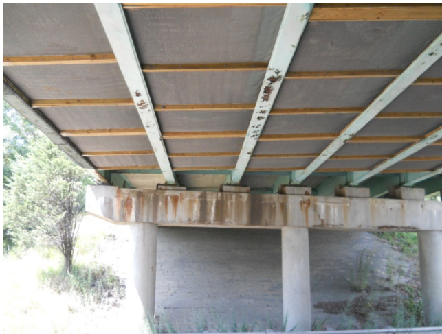
Figure 6: Debris netting under the SB Bridge
