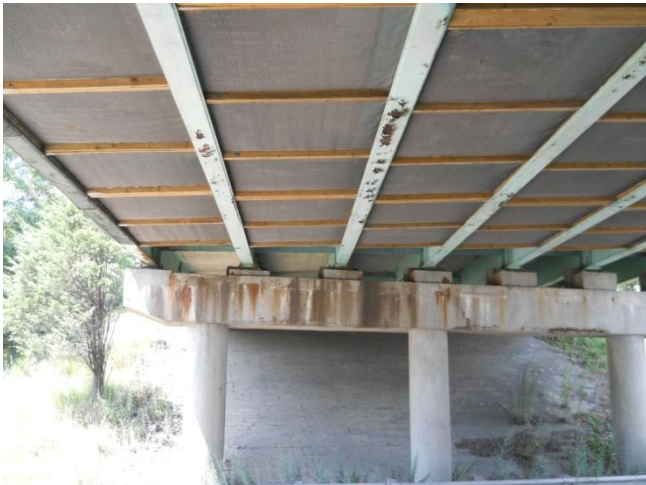
Figure 7: Debris netting under the SB Bridge
