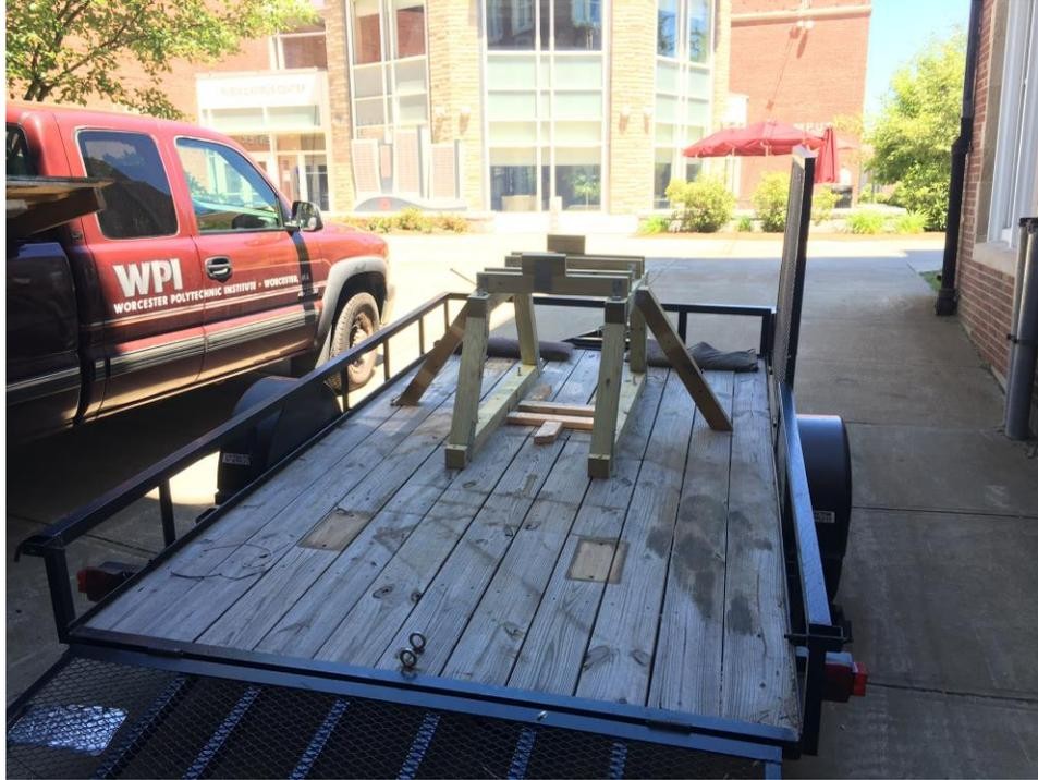
*Figure 37: Frame secured to trailer with added 45-degree supports*
