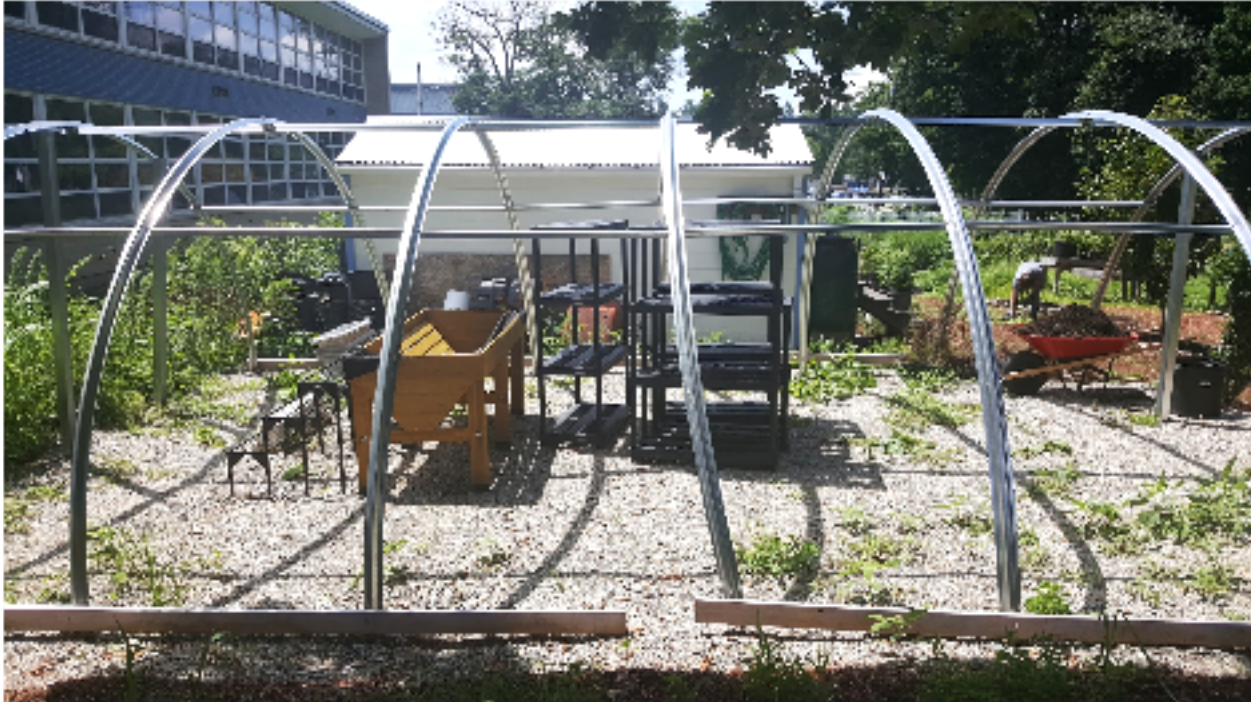
Figure 18: Unfinished Hoop House, Located Behind Storage Shed
