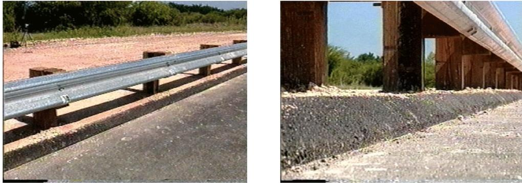
**Figure 2.10:** Guardrail/curb installation for TTI test 404201-1.(32)
