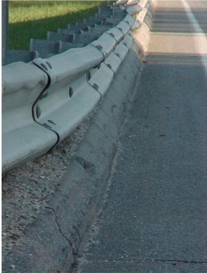
**Figure 1.2:** Sloping curb installed flush with a strong-post w-beam guardrail on a 90 km/hr two-lane rural roadway in Maine.
