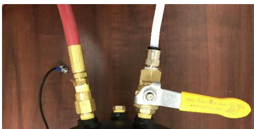
Figure 5A: Yellow valve handle perpendicular to air tank in the closed position
