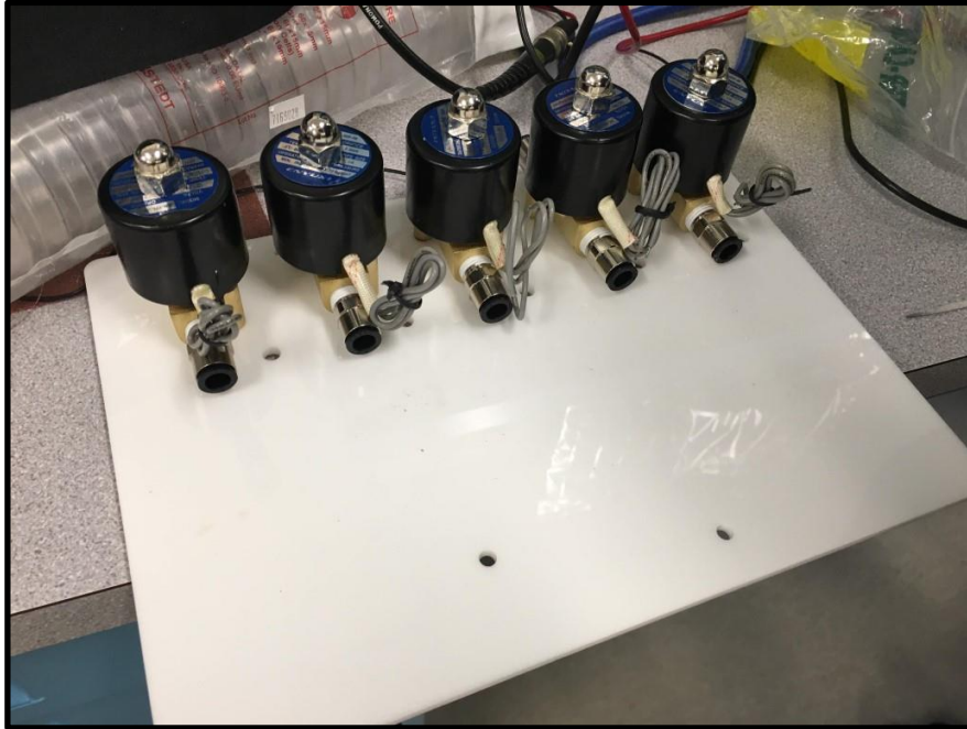
Figure 43: A picture of the top lid of the control panel which holds the solenoids in an array as depicted.
