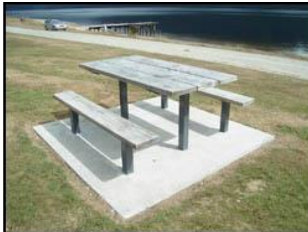
Figure 35: Table With Steel Frame Embedded in Concrete (Interempresas, 2015)
