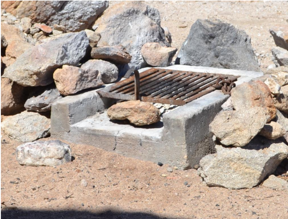
Figure 7: Braai Pit with Crack in Concrete Base
