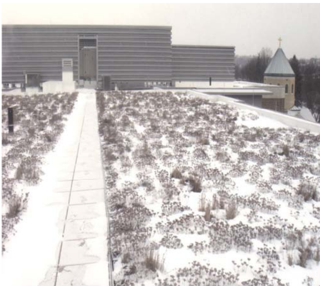
Figure 4.5: Green Roof, January 2010 (DiMauro)
