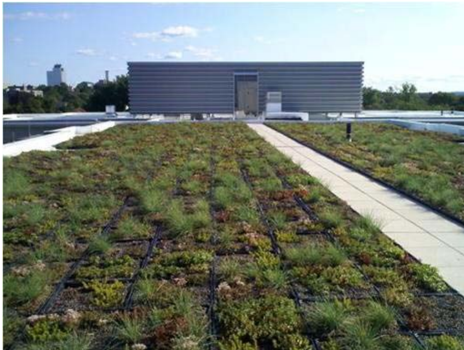
Figure 1.1: Nitsch/Maglioizzi Green Roof After Installation, August 2008
